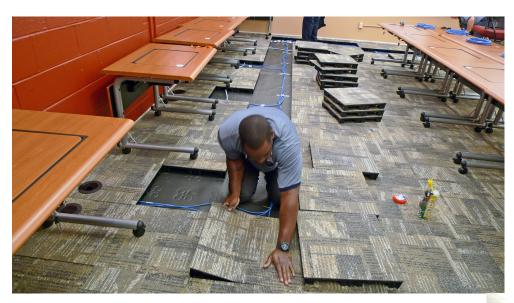
FITT Floor® carpeted panels are interchangeable, so outlets for power and data can be located and moved within the space. No special tools or electricians required for changes. UL Approved power connections, outlets and cables.
