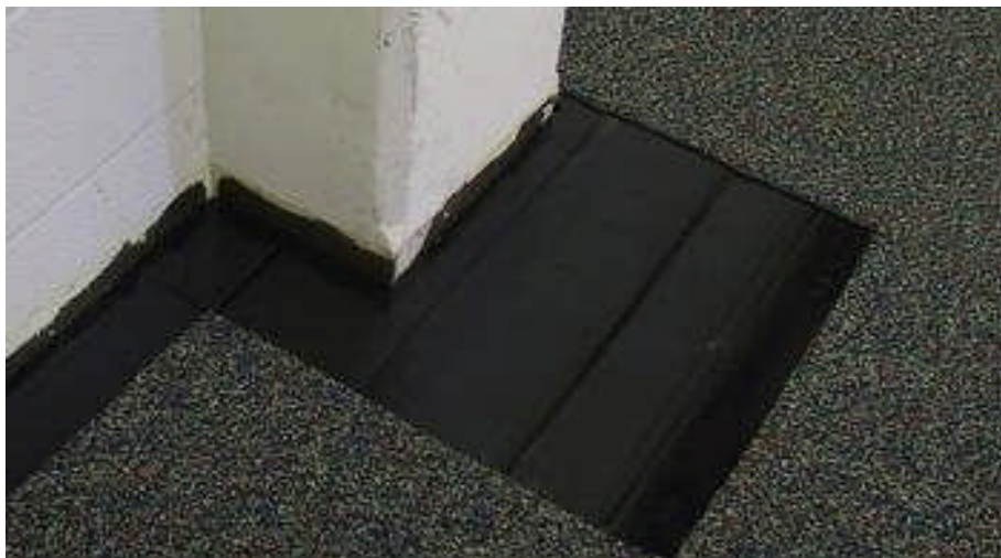
Picture 7-8 Filling in Perimeter around obstacles
