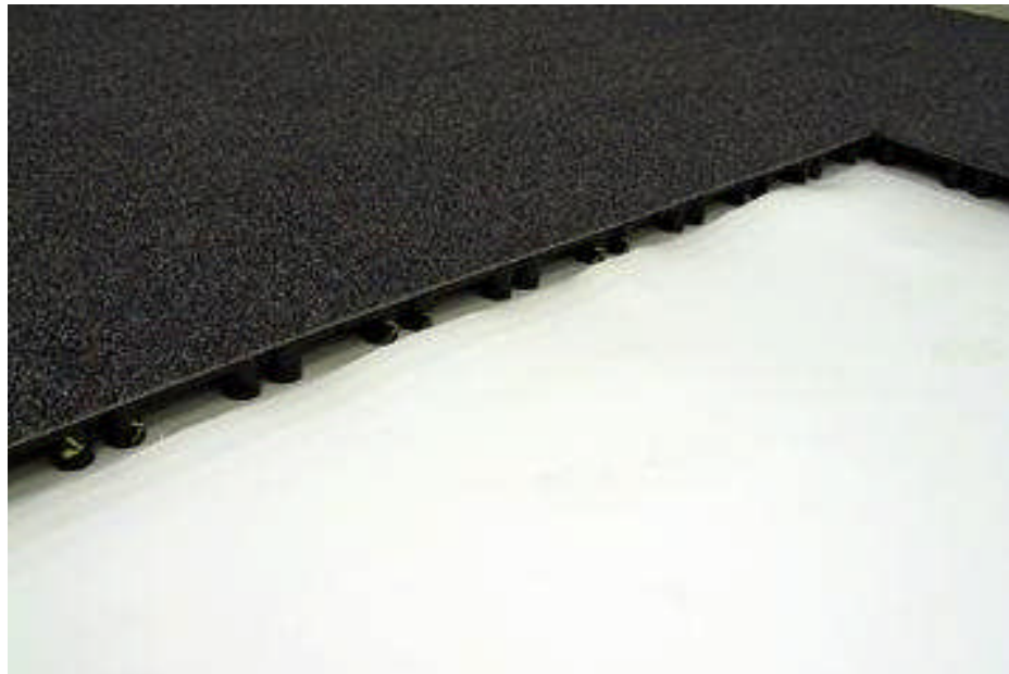
Installing Foam Underlay
