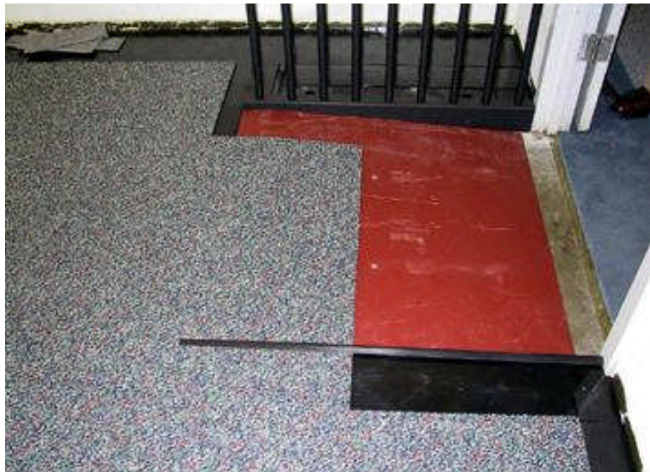
Carpet Tile seam installed beyond top and bottom of ramp
