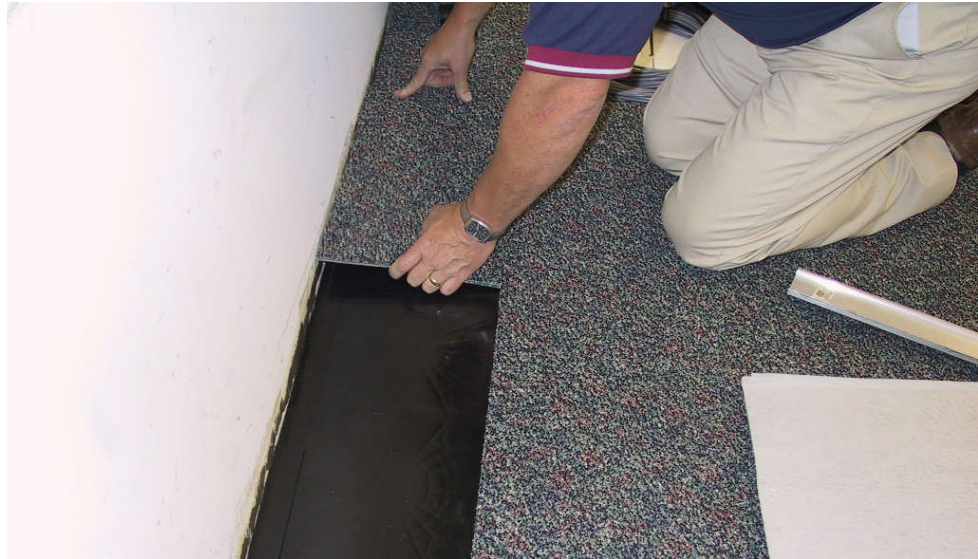
Installing carpet tile on perimeter
