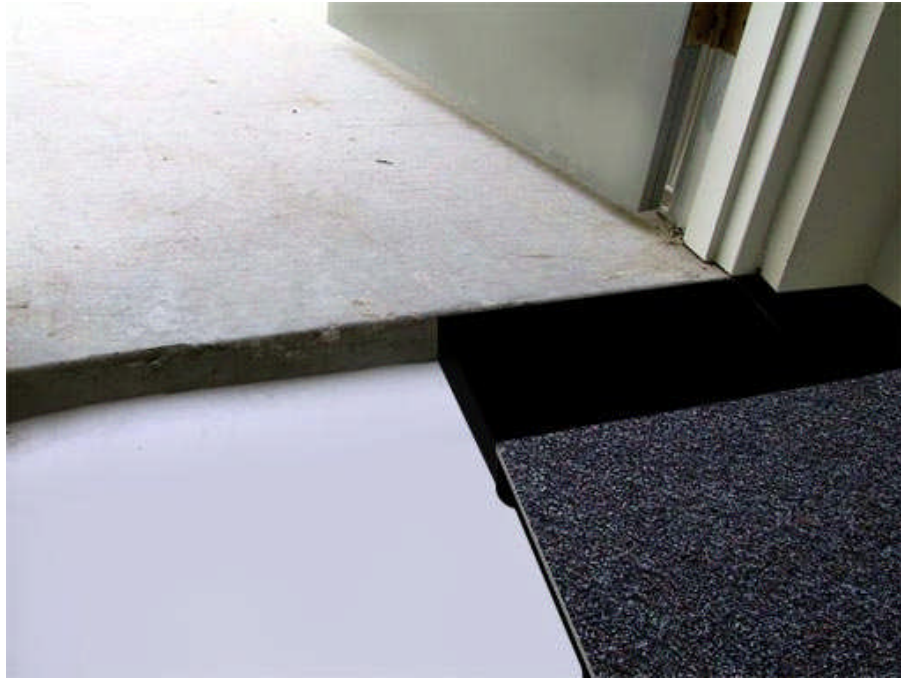
Picture 12-3 Recessed Sub-floor with full panels and perimeter filler installed
