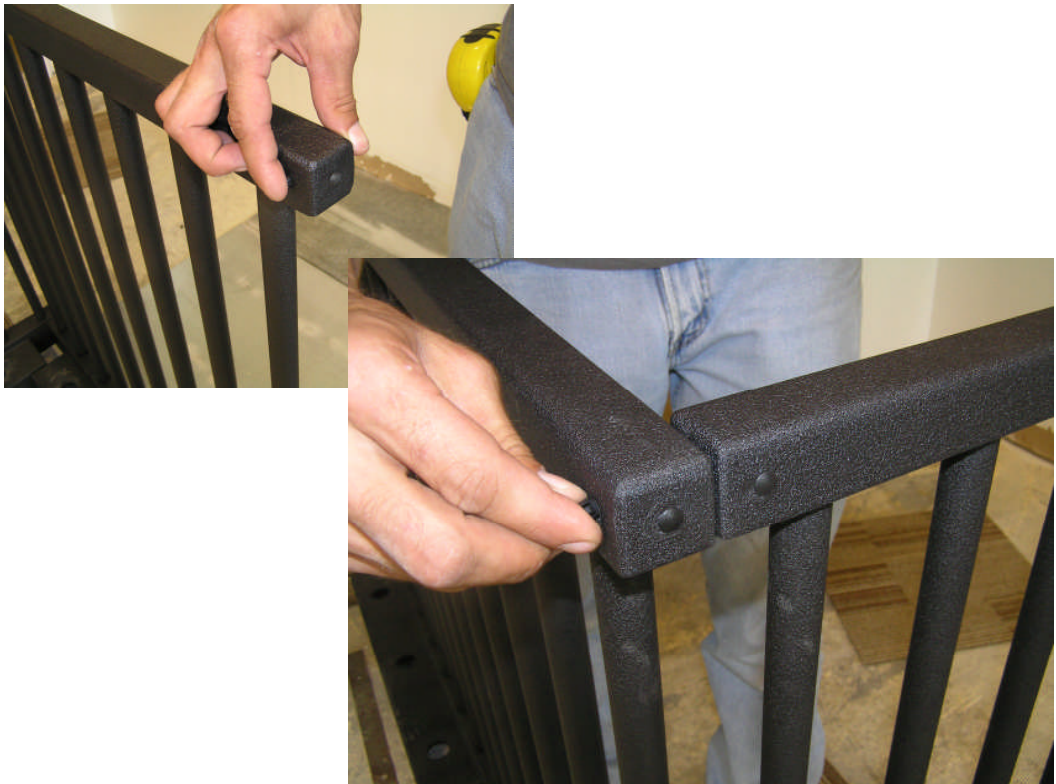
Picture 8-9 Rail Top Cap Holes are filled with Plugs
