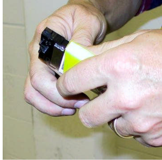
Picture 9-14 Applying Color Coding
