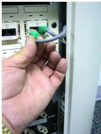
LDS with Patch Panels and Data Cables
