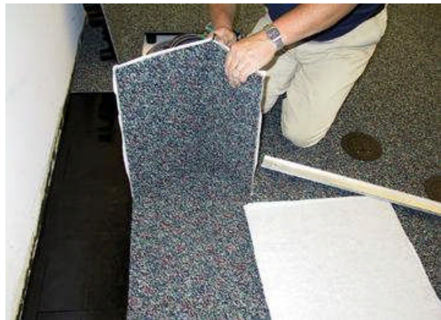
Cutting carpet tile for perimeter
