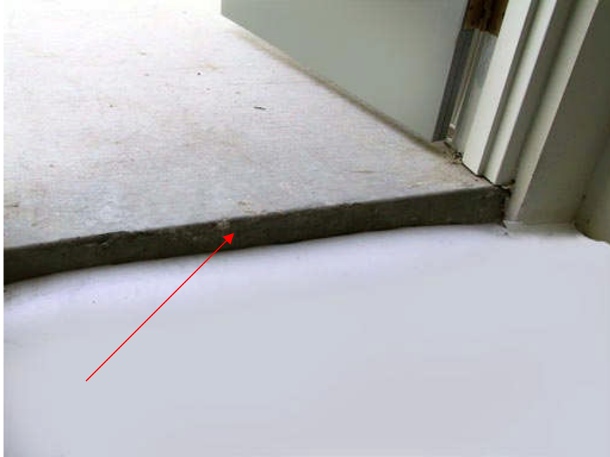
Picture 12-2 Recessed Sub-floor with full panels requiring perimeter filler
