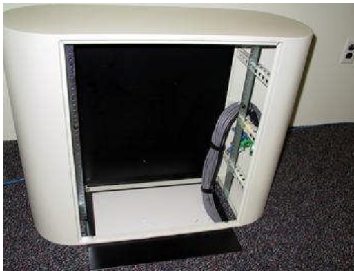
LDS with Data Cables fed through base
