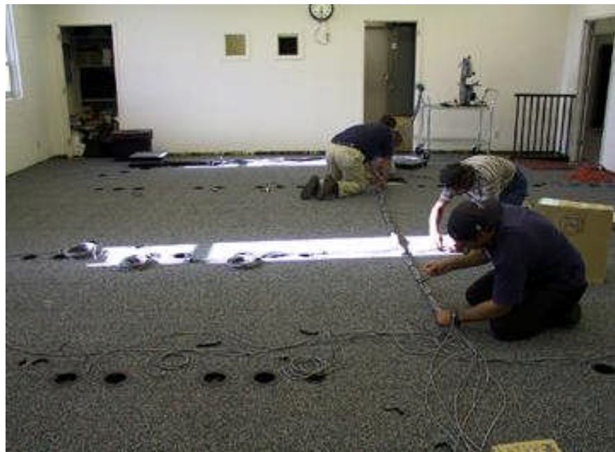
Tie Wrapping as Required
