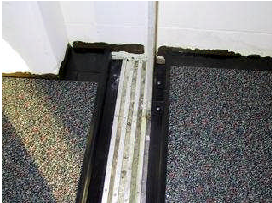
Picture 7-15 Z Trim Installed
