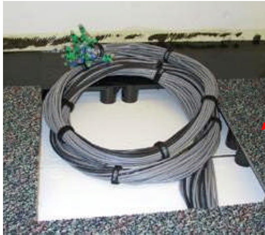
LDS with Data Cables fed through base
