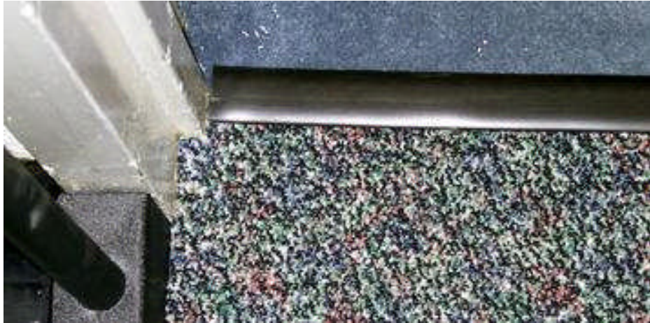
Installed Transition Molding
