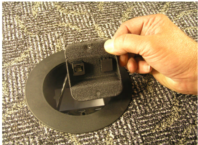
Mounting Plate is attached to Powerport
