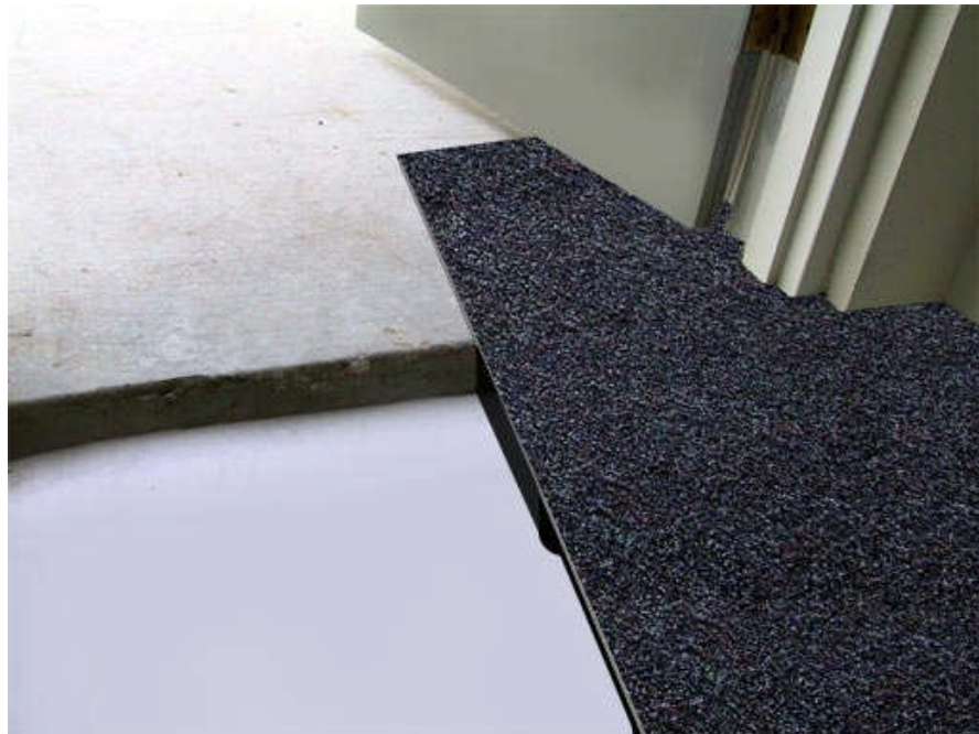
Picture 12-4 Recessed Sub-floor at Door Opening with full carpet tile overlaying perimeter and sub-floor seam
