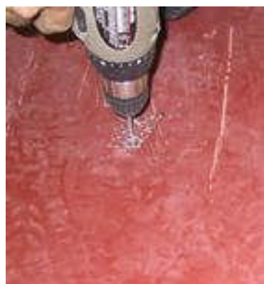
Drilling Ramp for countersunk anchors
