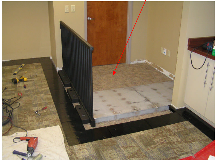
Drilling Ramp for countersunk anchors
