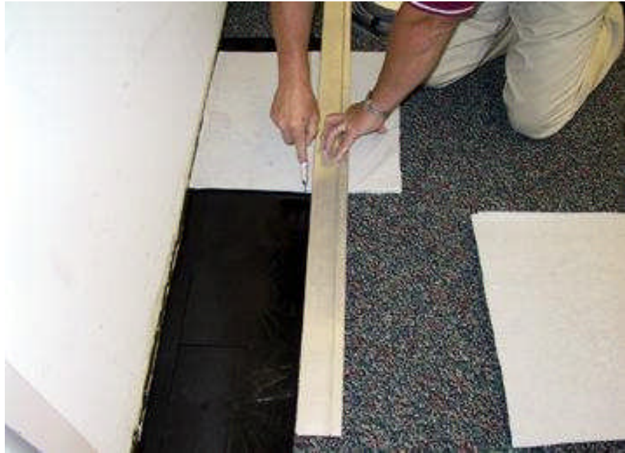
Cutting carpet tile for perimeter
