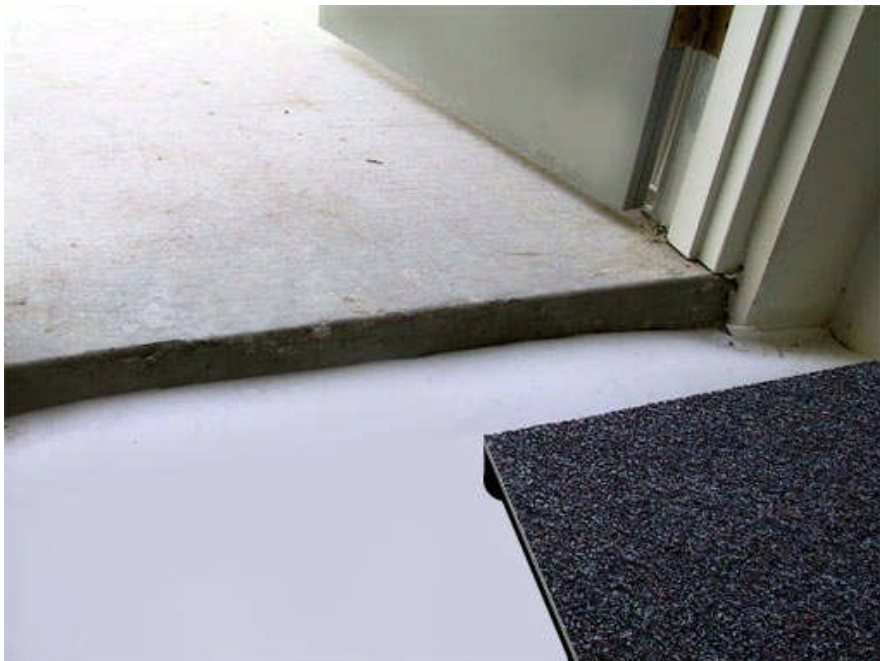
Picture 12-2 Recessed Sub-floor with full panels requiring perimeter filler
