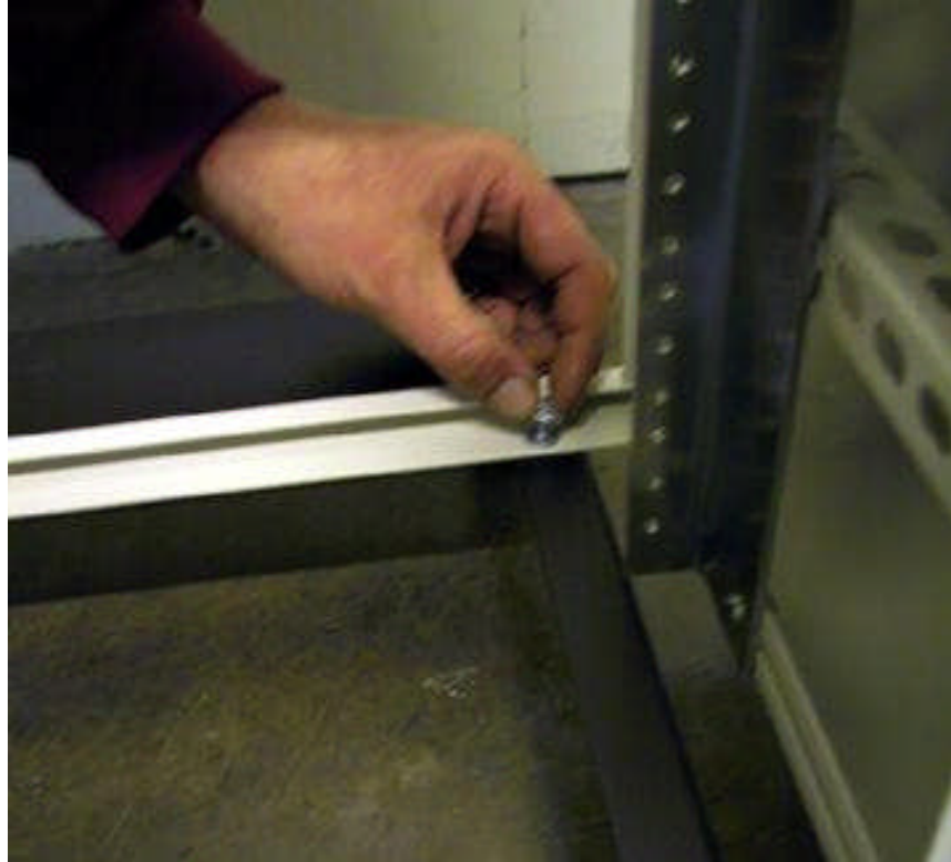
Picture 10-5 Installing LDS Cabinet to Base Unit
