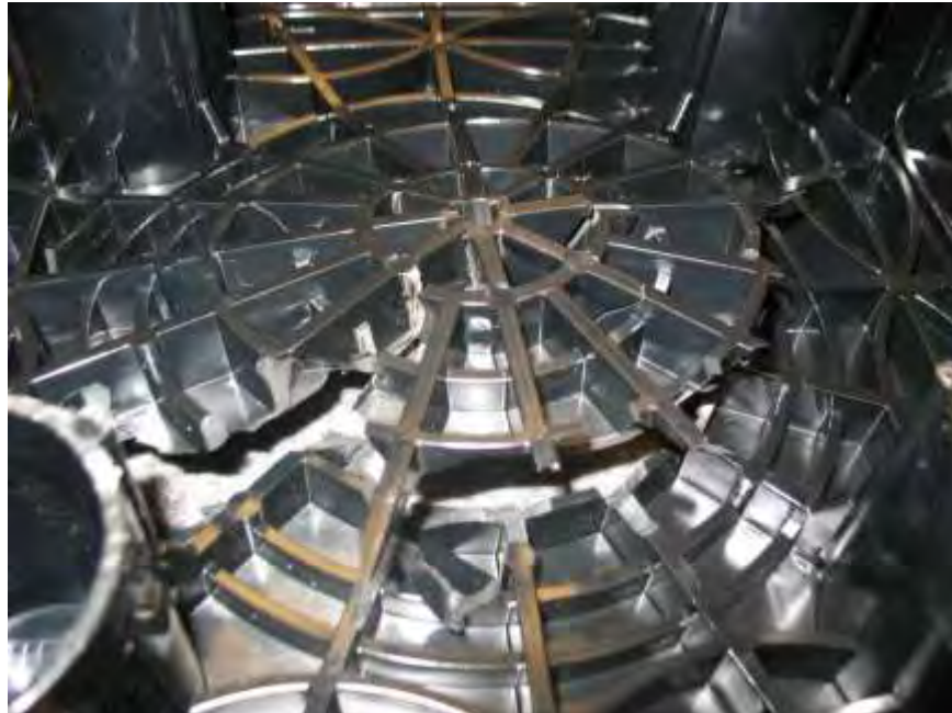
Photo No. 10 CISCA Sections 1 and 2 - Center of Quarter Panel Underside Failure Detail
