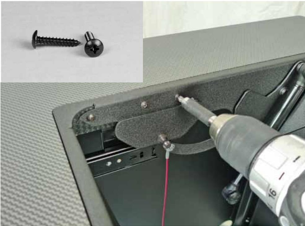
Six #2 Phillips drive wood screws are provided with the flipIT Kit for installing the collar. Three are installed in the left front side to provide added support for the pneumatic cylinder. The other three corners take one screw per corner.
