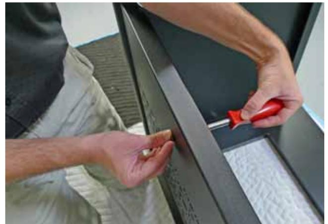
Use two machine screws with lock washers and nuts for installing the power strip to the modesty panel
