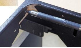
Lift the lid open all the way and complete the installation. One screw installs the right side corner. 3 screws reinforce the gas spring mounting post location on the left side.
