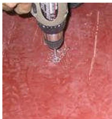
Countersinking the anchors used for mounting the ramps, eliminates any bulging in the carpet tile, placed on the ramp.
