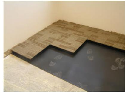
When starting the System at a corner with an obstacle, use three whole panels to determine the area around the obstacle. Corner area needs to be filled with appropriate perimeter / pedestal components and cut in around the obstacle, to provide a firm starting point.
