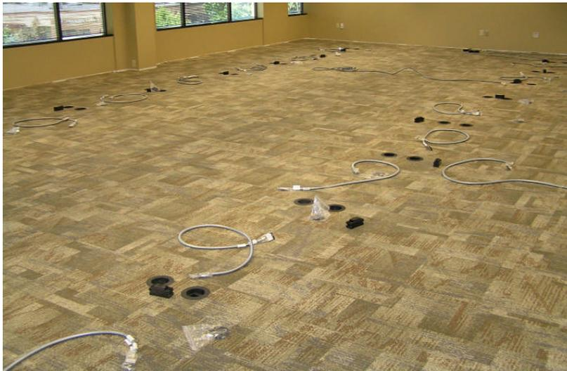
All cable assemblies & outlets can be plugged together, the cables can be color coded and a final check of layout can be made.
