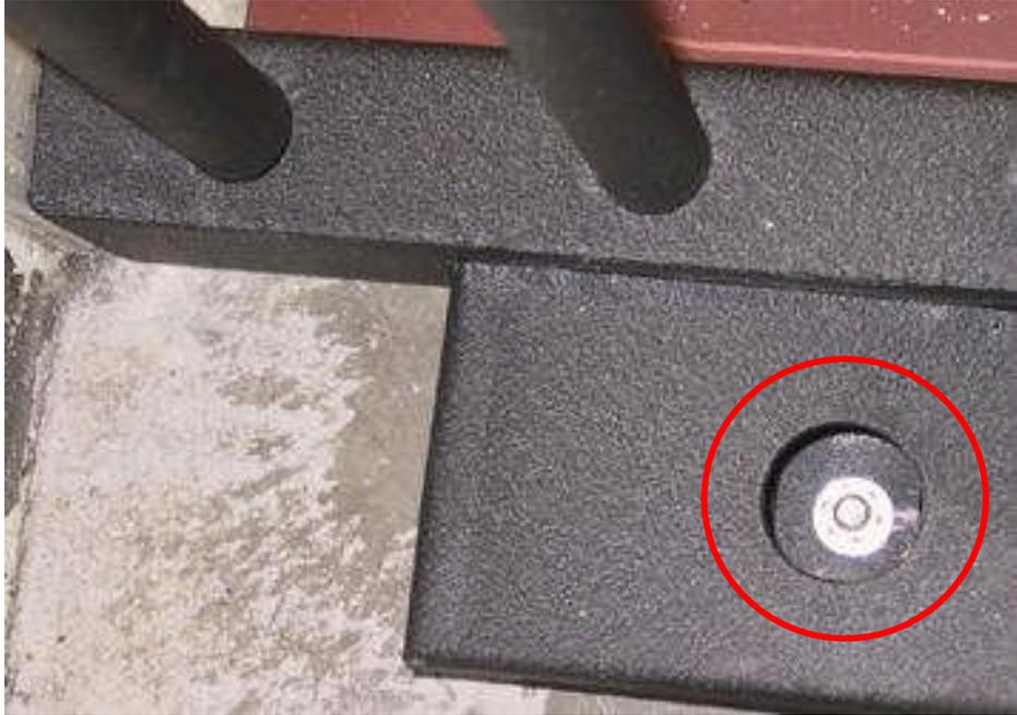
**Picture 8-9** Rail Top Cap Holes are filled with Plugs
