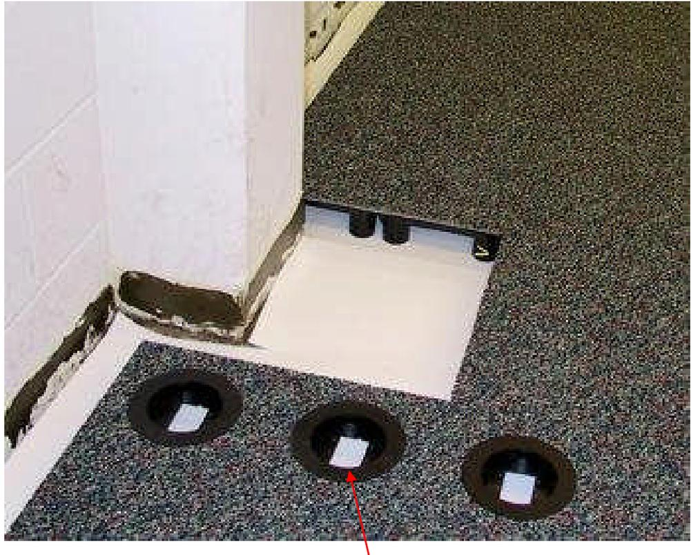
An appropriate quantity of whole panels will be supplied with outlet ports installed into them, per the project drawing. These outlet locations are provided with a universal outlet grommet ( **Powerport** grommet ) which is used for the installation of either electrical or communication components.
