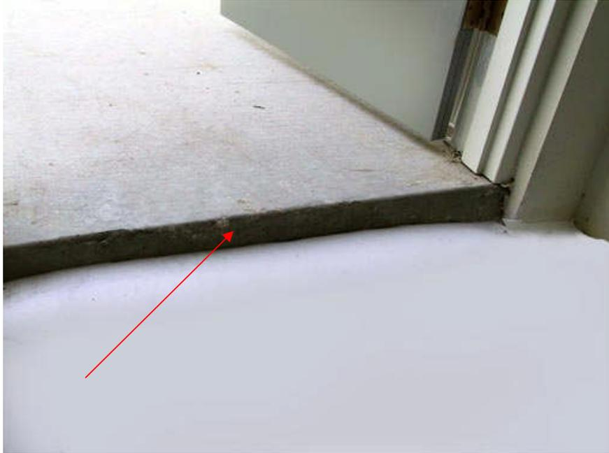
**Picture 12-2**      **Recessed Sub-floor with full panels requiring
