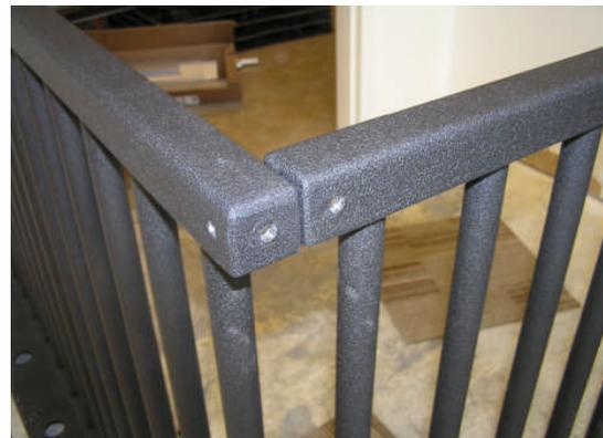
**Bolt is placed through the appropriate holes of the rail top cap, from the underside, and tightened.**
